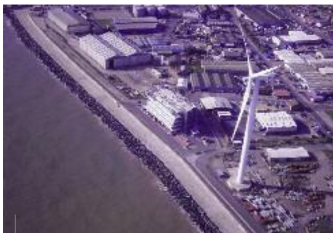
Aerial view over OrbisEnergy, Lowestoft
